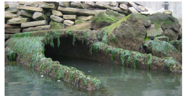
Combined Sewer Overflow outlets can also be a source of contamination. Challenges on land, include potential hydrocarbon soil contamination from the diesel tanks that used to sit on the site, in addition to the fact that the whole site is unengineered fill..
