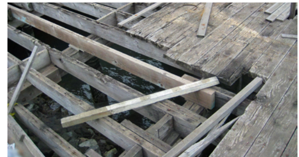
The wharf is structurally unsound, and the piles and beams have been treated with creosote.
