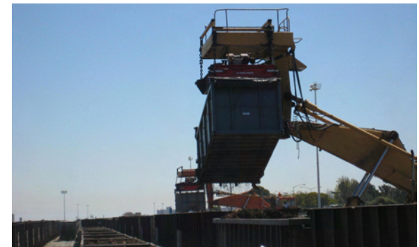
Contaminated soil deposited into SFBR aggregate gondolas
