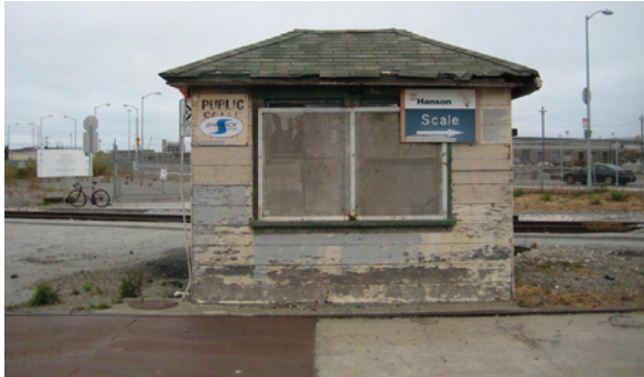
A potentially historic scale house, once used to weigh freight trucks, sits on the site.
