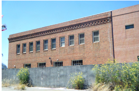
There's an 8' plywood fence around 3 sides of the firehouse. The firemen want to protect their privacy.
